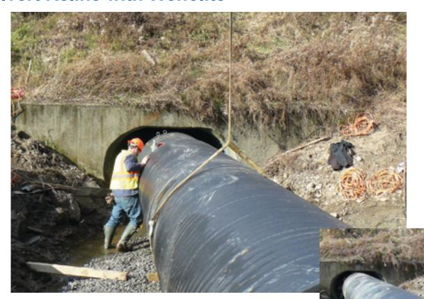
In 2007, NYDOT Region 9 turned to Weholite for assistance with an emergency culvert slipline under deep fill. Based on success of that project, Region 9 once again turned to Weholite for a long lasting, economical solution to some deteriorating culverts under deep fill.
